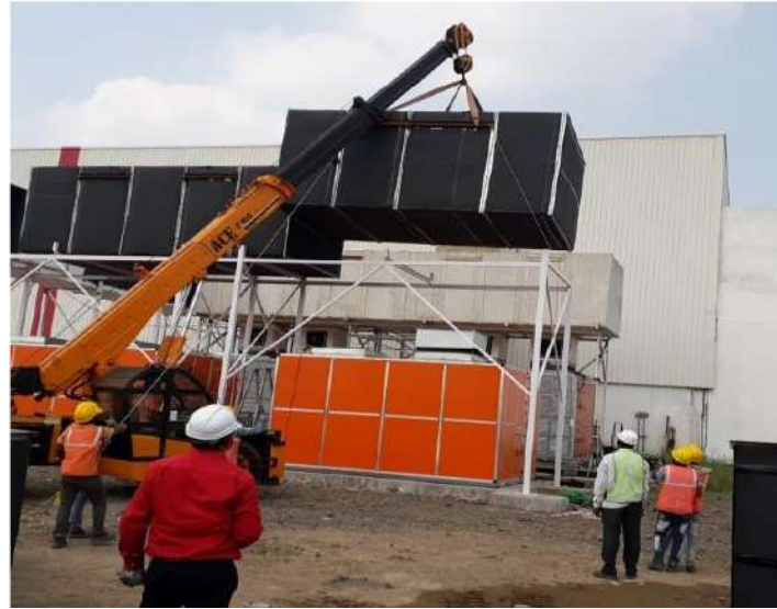
Duct Plenum Lifting
