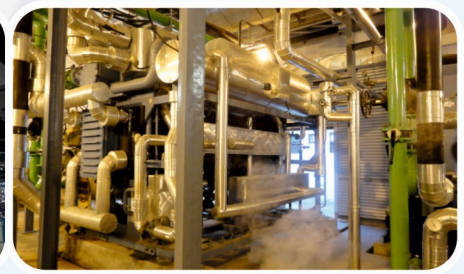
Project @ Anantara, Maldives
